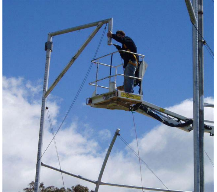
JUST COULDN'T KEEP EVAN ON THE GROUND, NOT SURE WHAT IS WITH HIM AND HEIGHTS, THIS TIME DRILLING THE GATE FOR THE I BOLT FOR THE GATE PULL ROPE.
