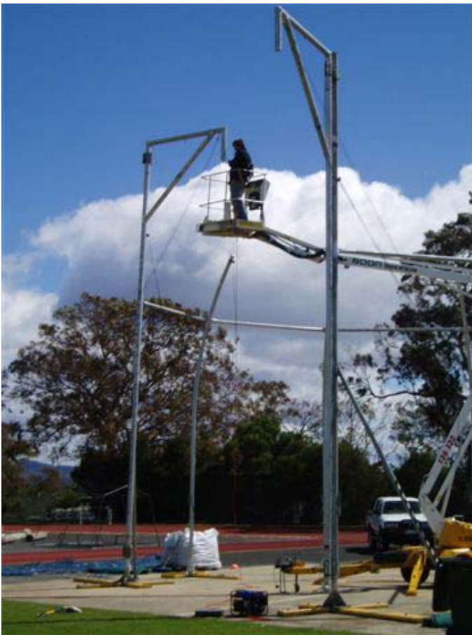
JUST COULDN'T KEEP EVAN ON THE GROUND, NOT SURE WHAT IS WITH HIM AND HEIGHTS, THIS TIME DRILLING THE GATE FOR THE I BOLT FOR THE GATE PULL ROPE.
